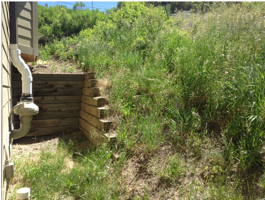
Existing wall to be extended into the foreground of the photo.
