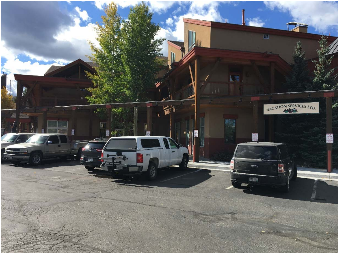
PZ21-19, Series of 2019 Master Sign Plan Amendment for the Durango Court Building Existing Conditions
